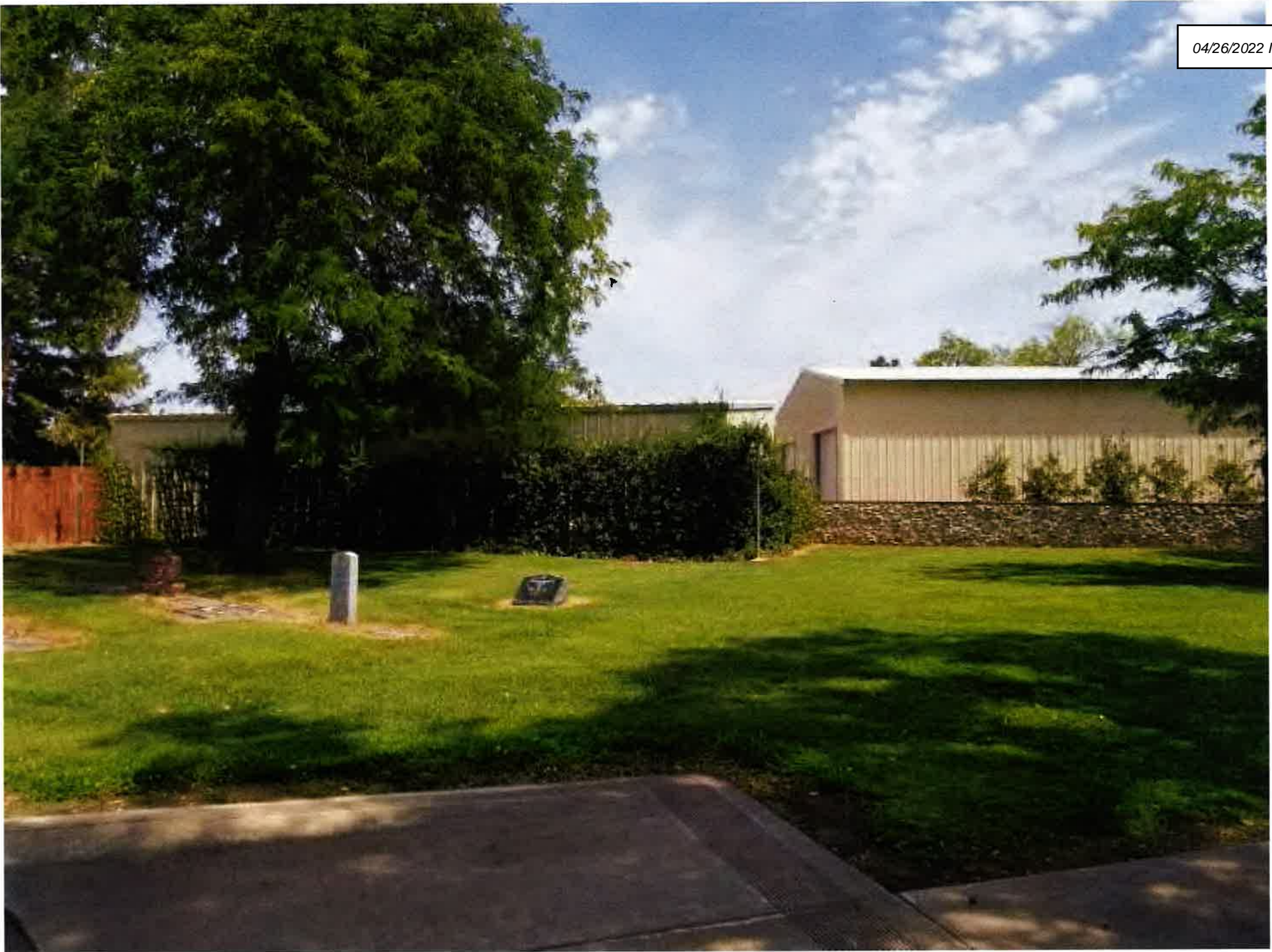
VIEW OF MAINTENANCE AREA FROM INSIDE CEMETERY
