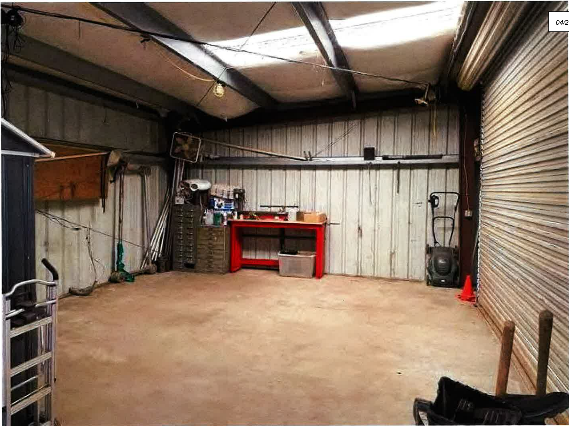
VIEW INSIDE STRUCTURE FOR PROPOSED CREMATORIUM
