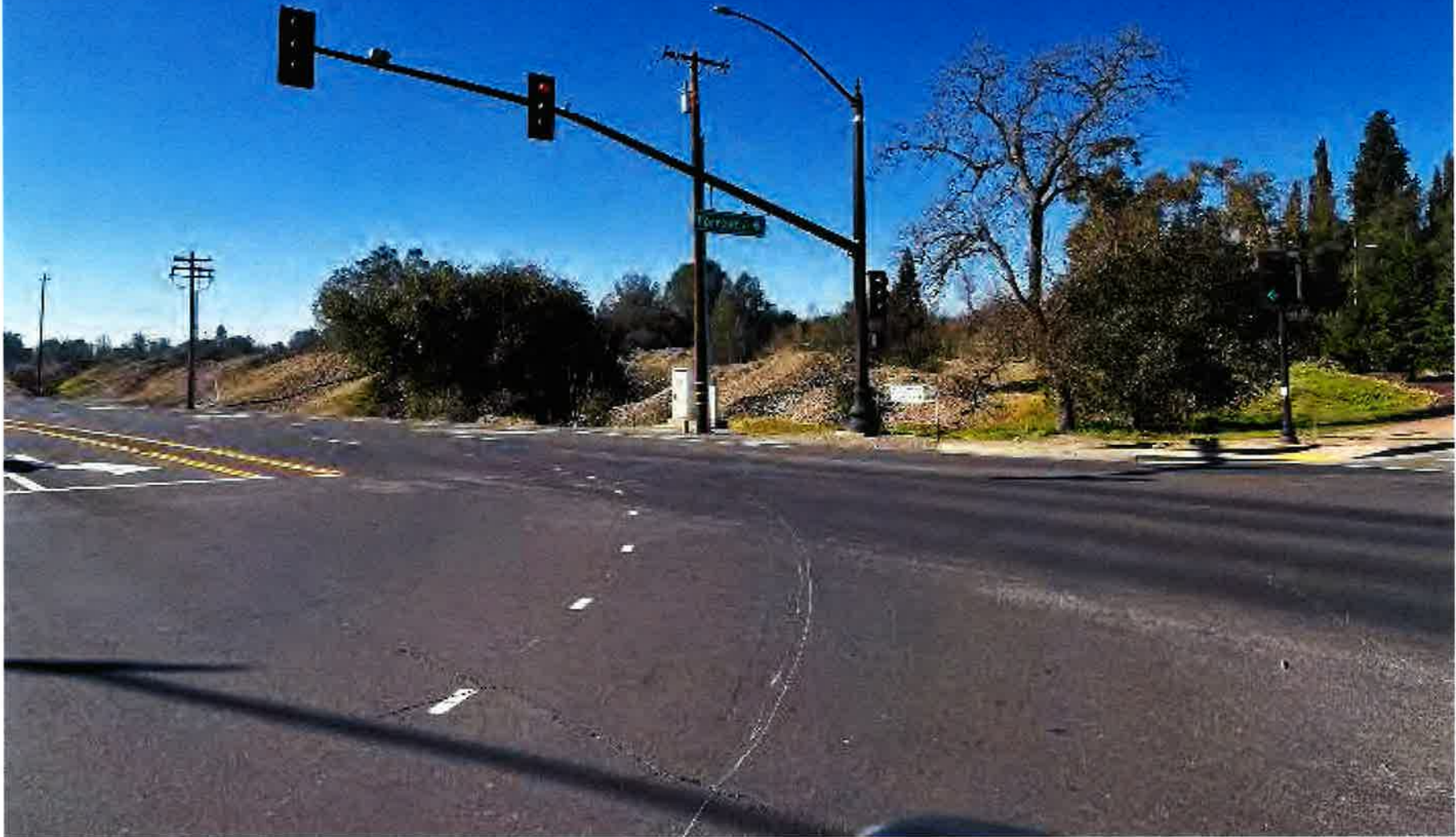
VIEW OF MINING TAILINGS FROM FOLSOM BOULEVARD AND FORREST STREET
